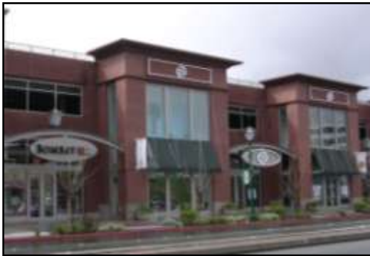
vertical articulation treatment (min. 12" in width), color texture or material change
